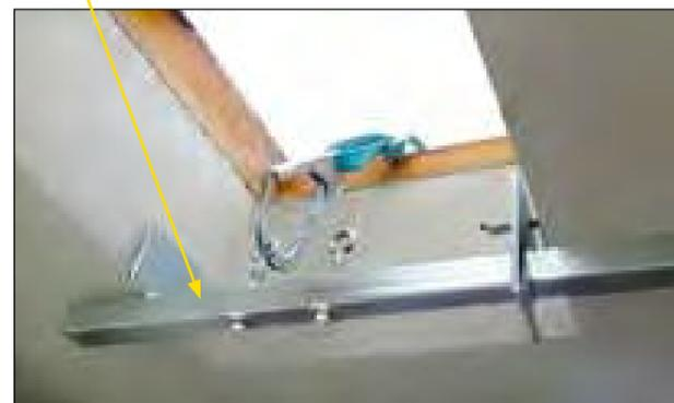
**BARRA DI ANCORAGGIO REGOLABILE PER INFISSI UNI EN 795 CLASSE B**
